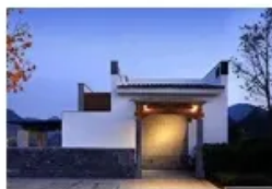
Household Energy Storage
