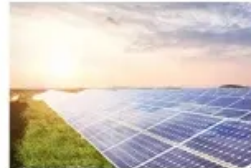
Energy Storage System
